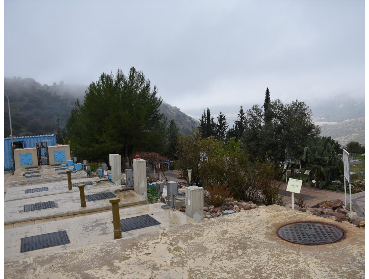
Demonstration; various systems in one location
